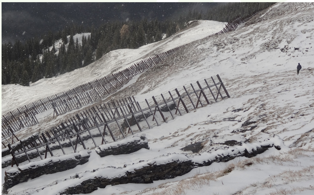
Picture 29. Structural measures and forest protection against avalanches.
