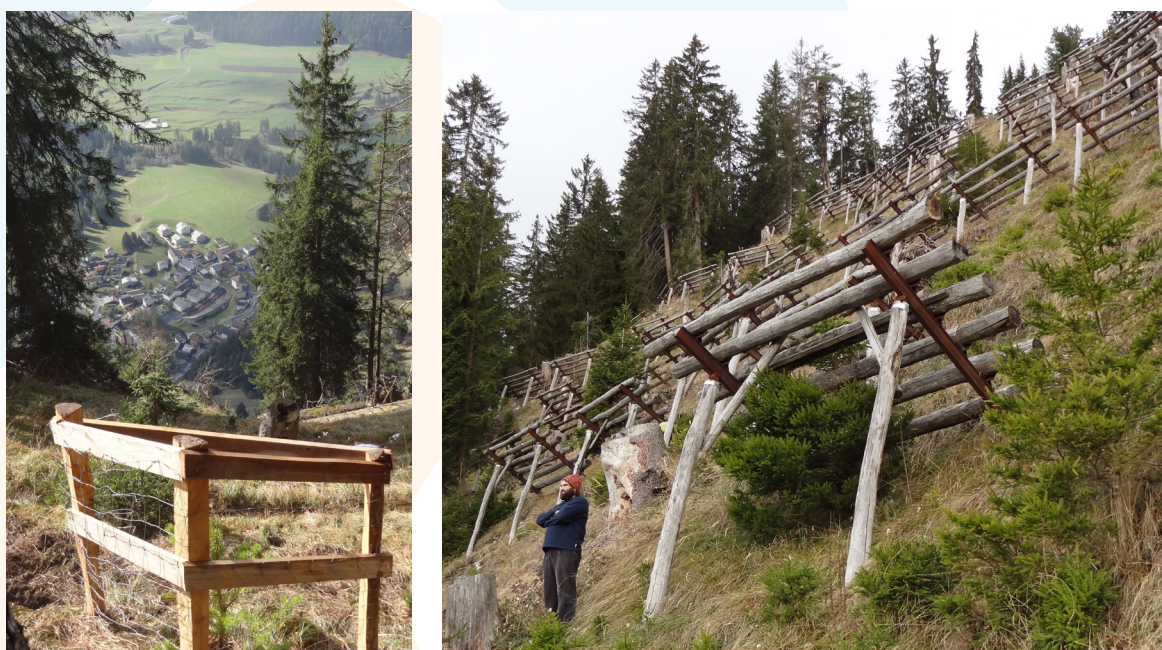
Picture 33 and 34. Temporary protection measures to recover an Alpine coniferous avalanche protection forest affected by a wildfire in the municipality of Trin (Switzerland).
