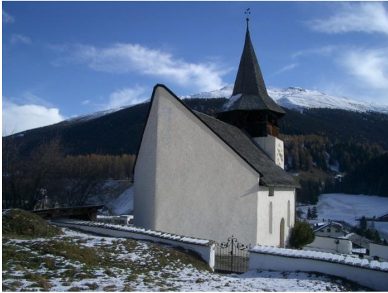
Frauenkirche Davos: A protection-wedge has been built after an avalanche destroyed the church in 1602
