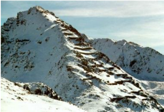
First technical measures, built around 1900
