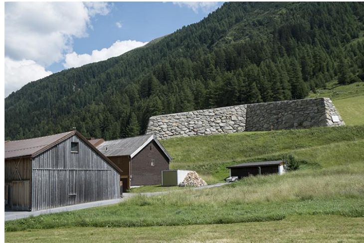
Stone wall (Galtür, Austria), built after Avalanche catastrophe in 1999
