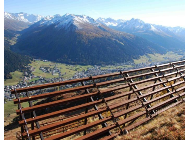
Avalanche barriers made of steel (after ca. 1950)
